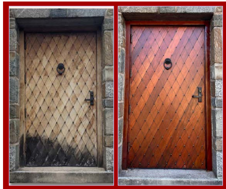
Library Door before & after refinishing
