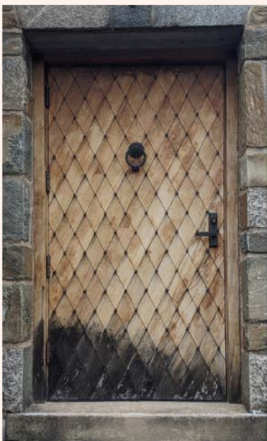
Library door before removal for refinishing work.
